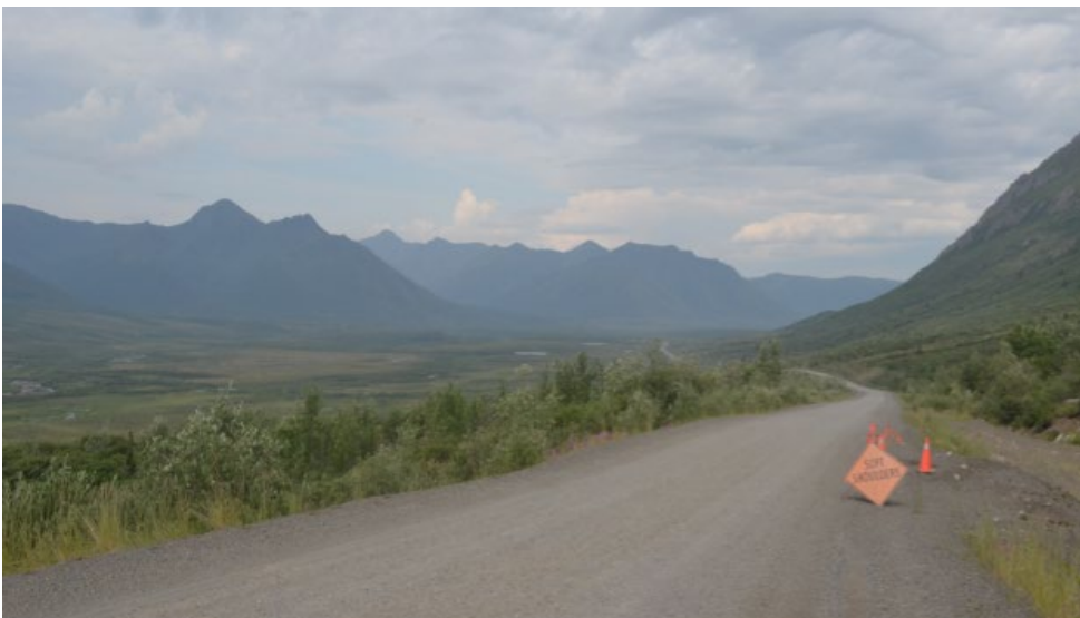
Dempster Highway north of Eagle River bridge (top) and in the Ogilvie River Valley (bottom).
